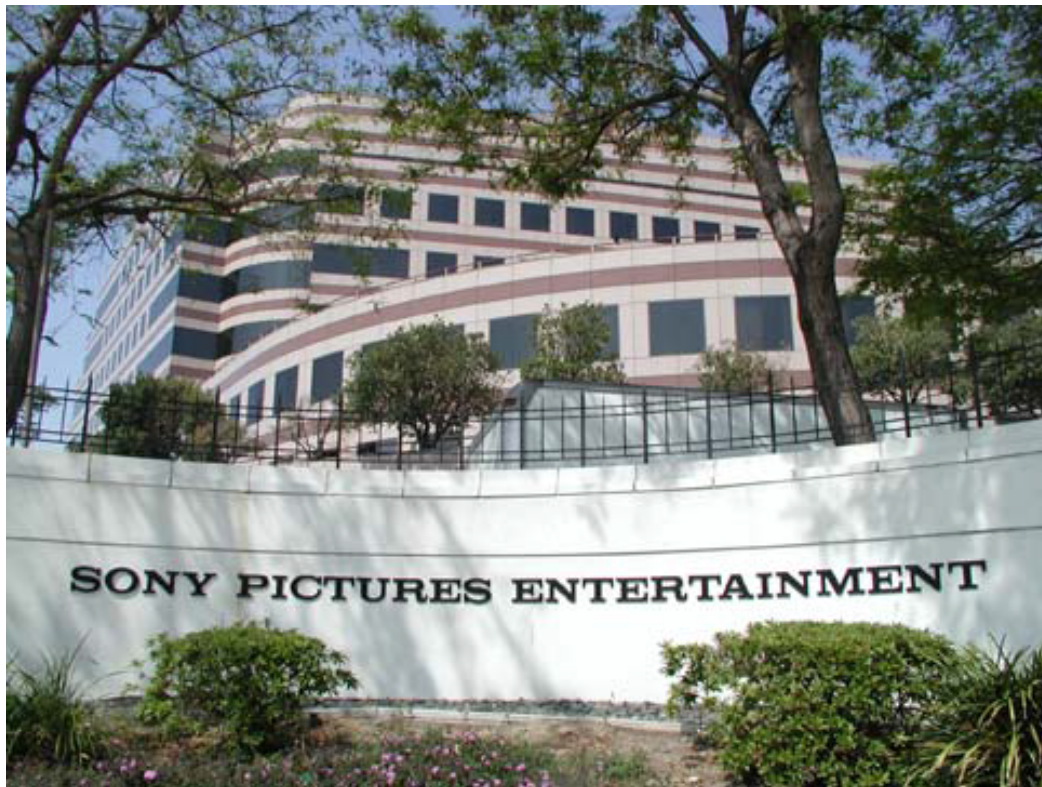
Figure 50. Sony Pictures Entertainment Located on Culver Boulevard.
