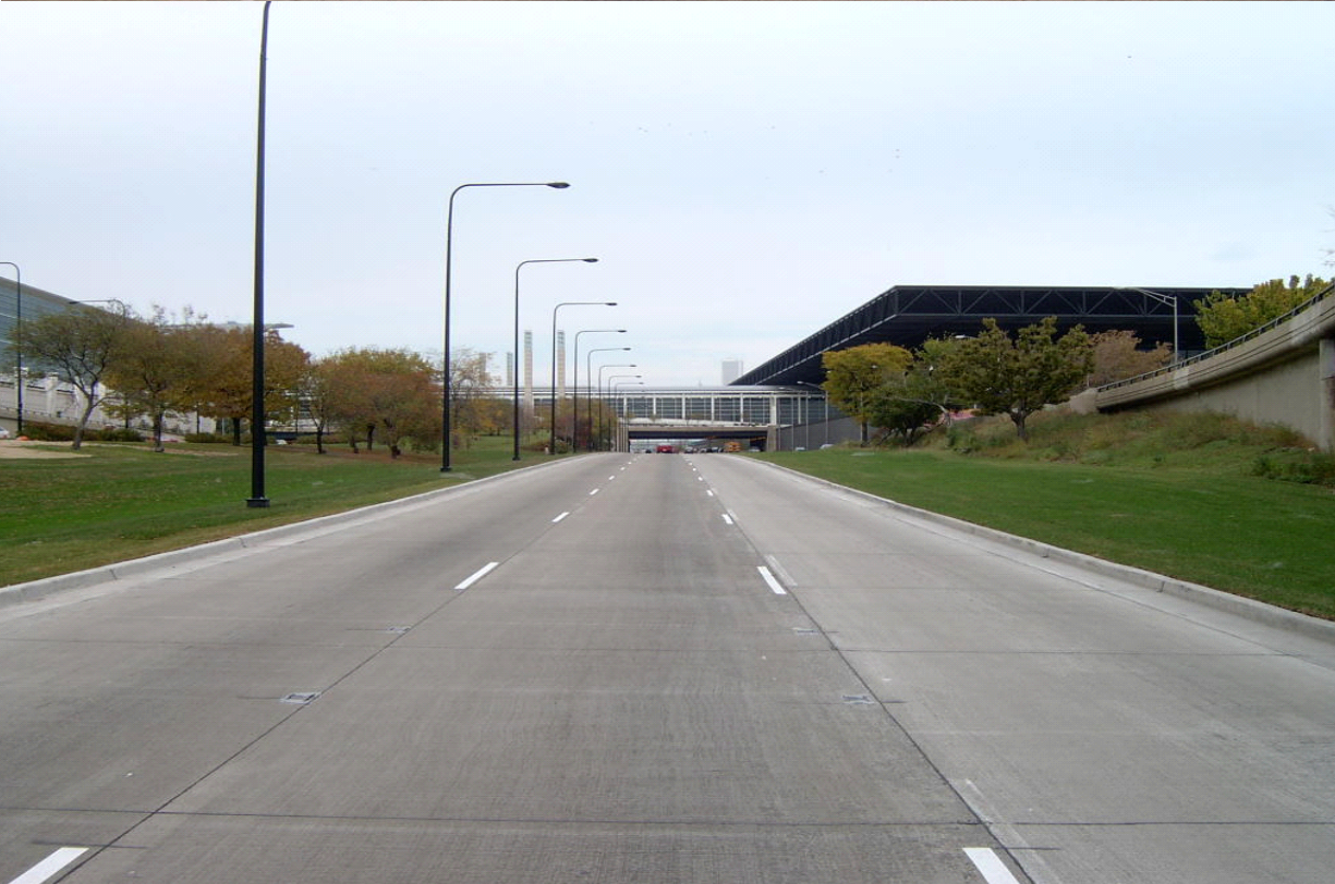
Figure 45. Before and After Photos of SLSD Depicting the Elimination of Shoulders and the Narrowing of Vehicle Lanes along SLSD Source: City of Chicago et al.
