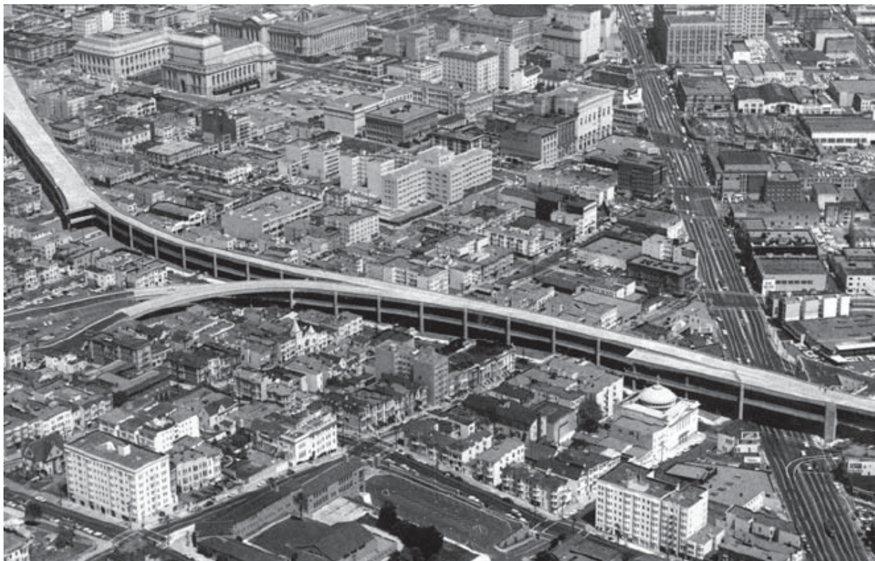
Figure 55. The Former Central Freeway with Market Street on the Left and the Connector to the Fell-Oak Pair Veering Off to the Left.
