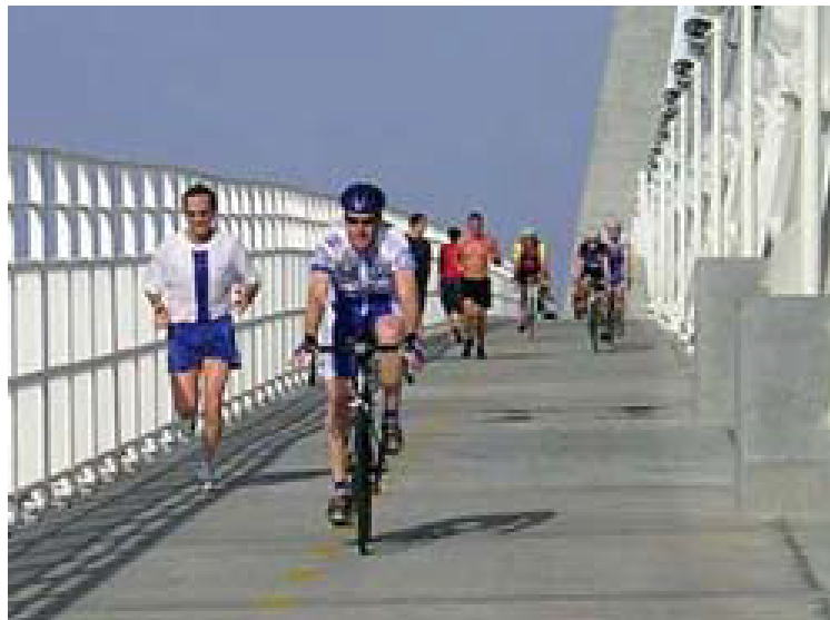
Figure 19. Pedestrian and Bike Path Spanning the Cooper River Bridge.
