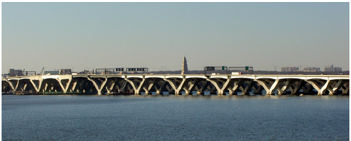
Figure 35. Image of the Completed Portion of the Woodrow Wilson Bridge.
