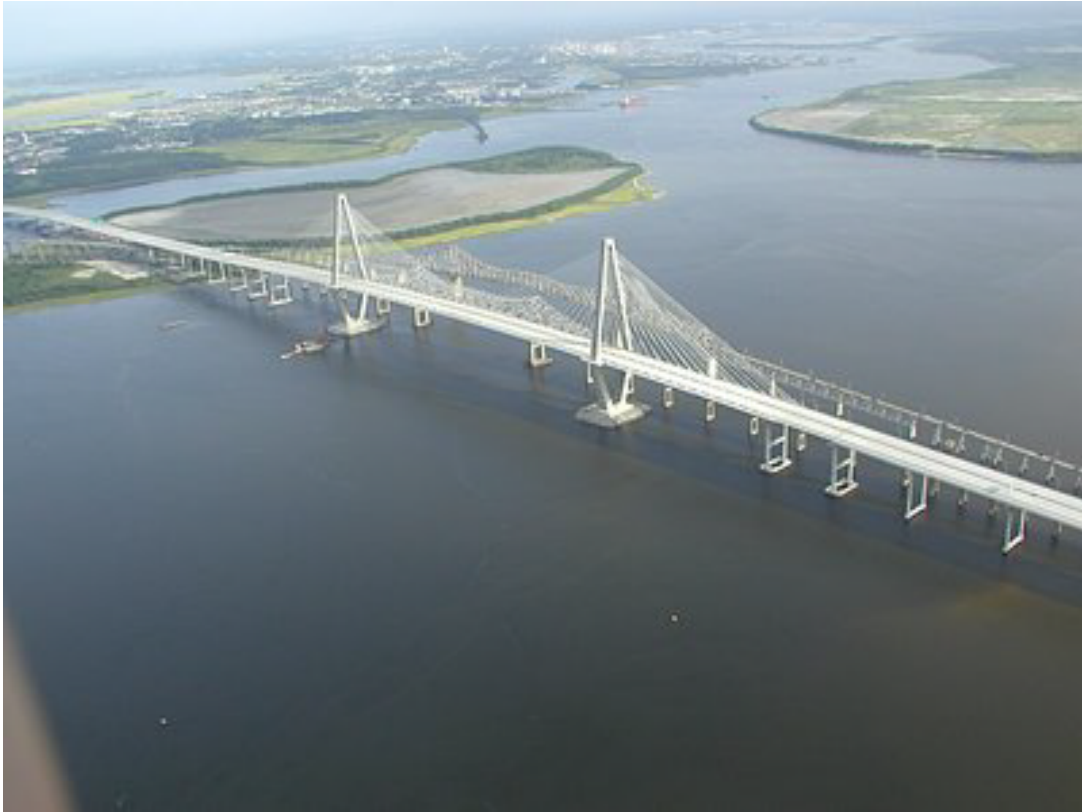
Figure 18. Cooper River Bridge Overhead Showing the Diamond Cable-Stay Design.
