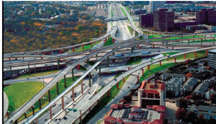
Figure 10. Completed I-635-US 75 (High Five) Interchange.
