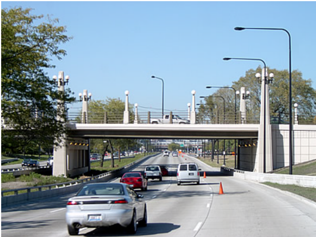
Figure 44. 31 st Street Bridge.
