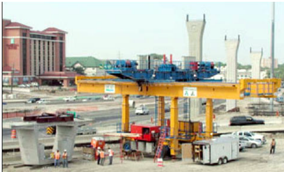
Figure 9. Segment Erector Technology.
