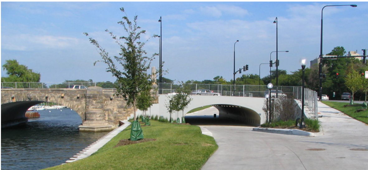
Figure 42. Marquette Underpass Source: City of Chicago et al
