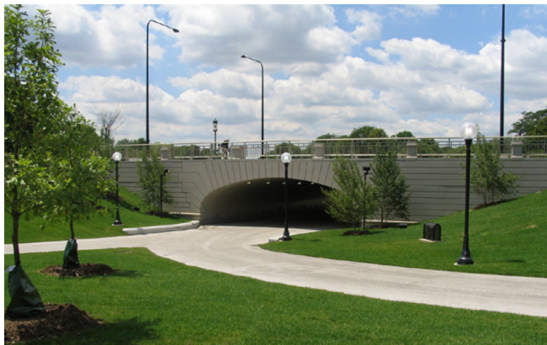
Figure 40. 59th Street Underpass Source: City of Chicago et al.
