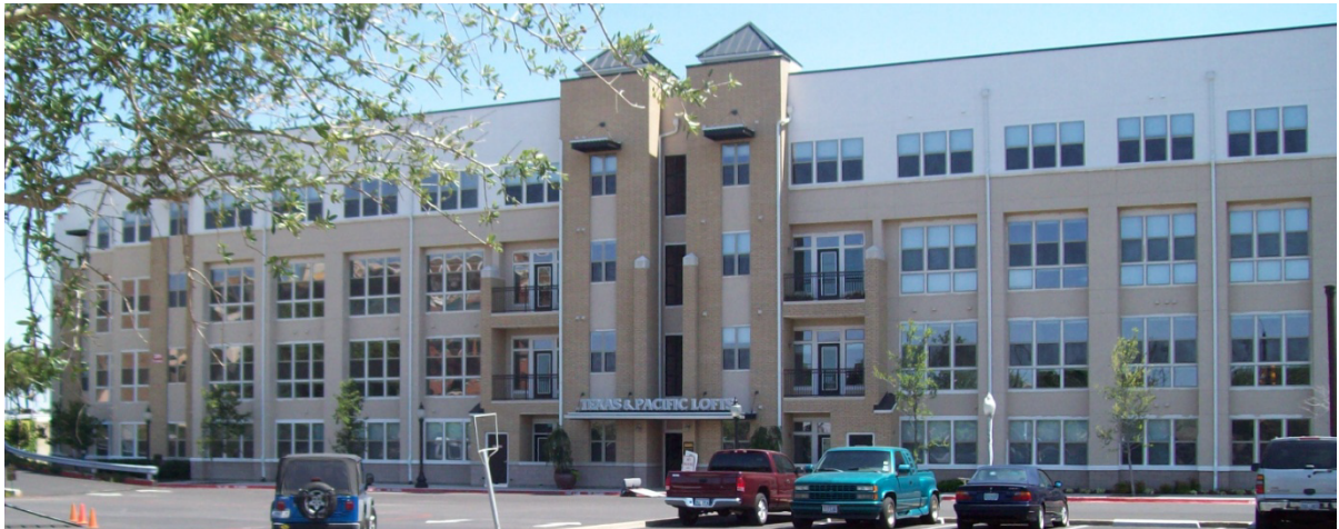
Figure 3. New Lofts Building Next to Old T&P Railroad Station Building. Source: Texas Transportation Institute
