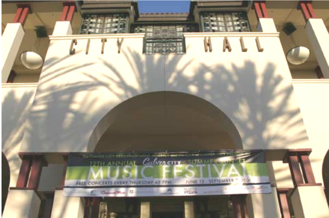
Figure 54. Culver City Hall's Movie Studio Type Façade. Source: http://www.culvercity.org/info/harry_culver.asp?sec=arts
