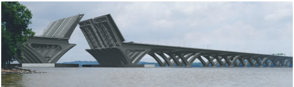
Figure 34. Image of the Completed Portion of the Woodrow Wilson Bridge.
