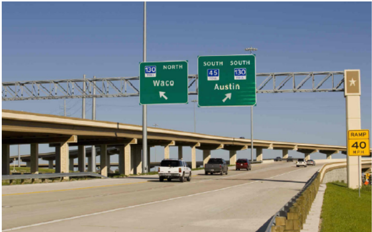
Figure 12. Appearance Features on Bridge and Sign Structures.
