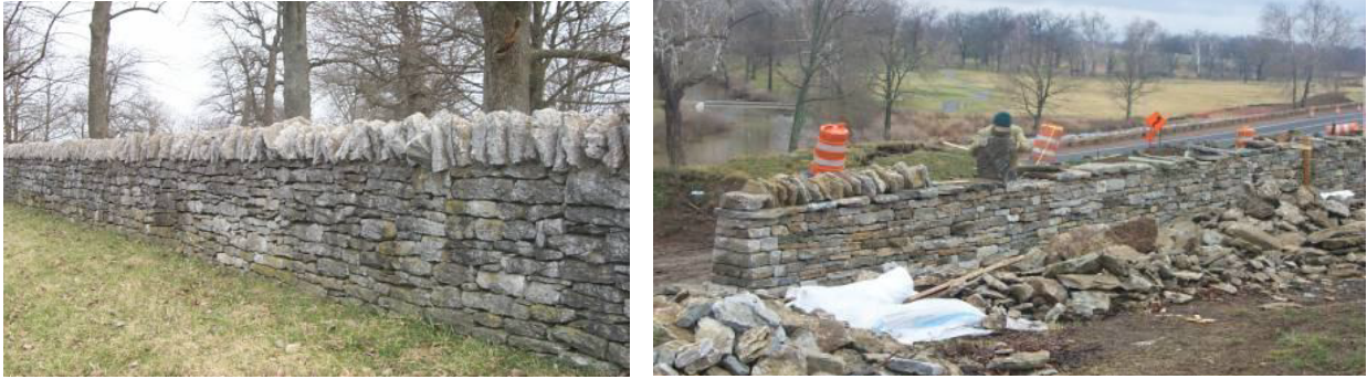
Figure 27. Historic Dry-Stone Walls Preserved or Re-Fabricated during the Paris Pike Project.
