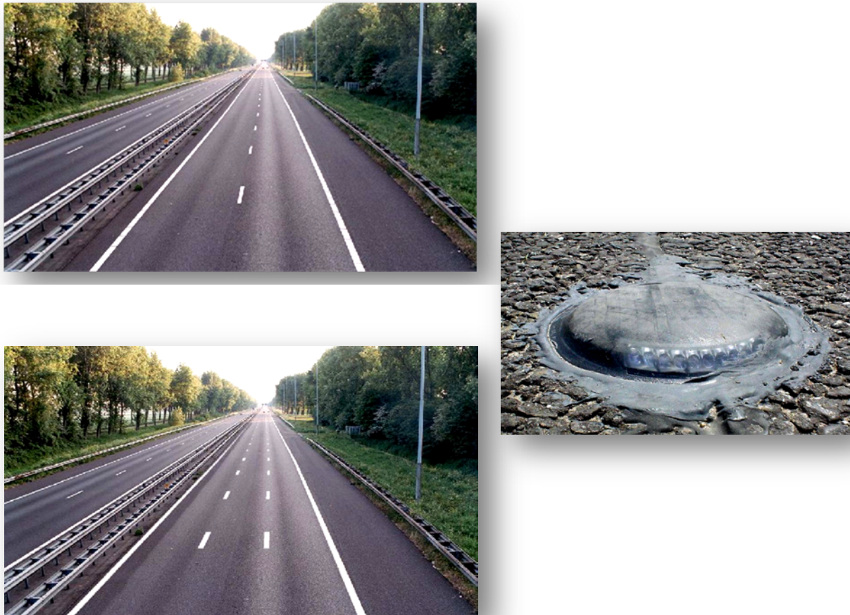
Figure 7. Left, a “flexroad” with its two possible cross sections on the A44. Right, an LED-based pavement device used for dynamic lane marking (8).
