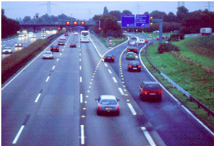
At an Exit with Hard Shoulder Running, The Netherlands ( PB )
